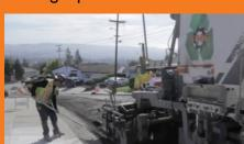
design specifications and mixed with a recycling agent and/or binder in the machine's heavy duty chamber before it is put down on the same road. The new mix is spread uniformly across the road by the machine's
